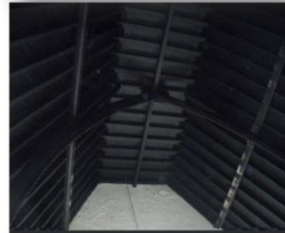
Figure 1 – inside view of existing roof
